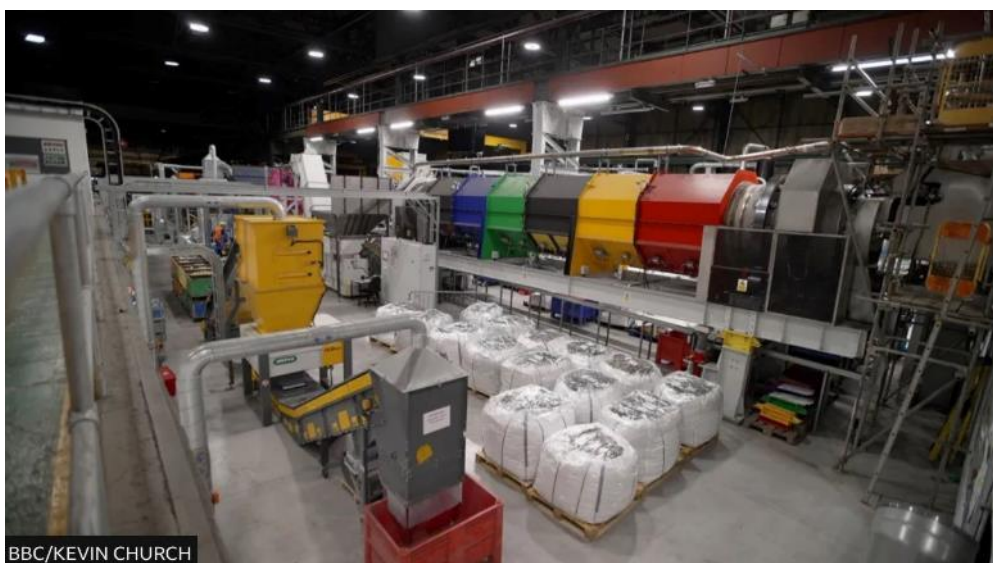
The Royal Mint reclamation plant
